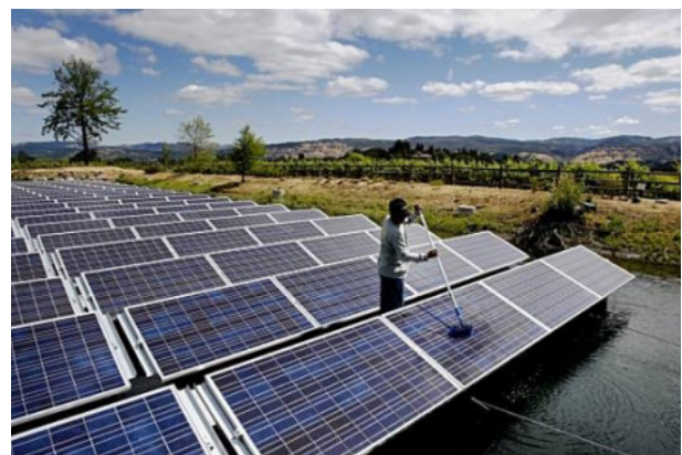
Photovoltaic installation in Ethiopia (Image: BPVA.org)
