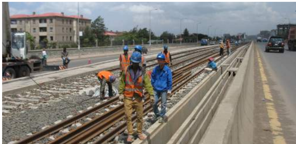
Construction of the light railway in Addis Ababa
