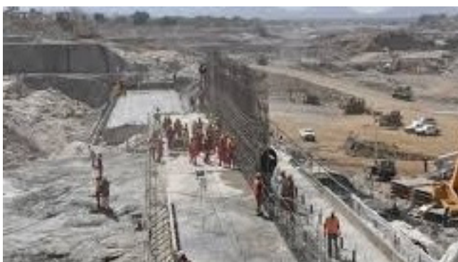
Construction of the Grand Ethiopian Renaissance Dam, 42 percent completed
