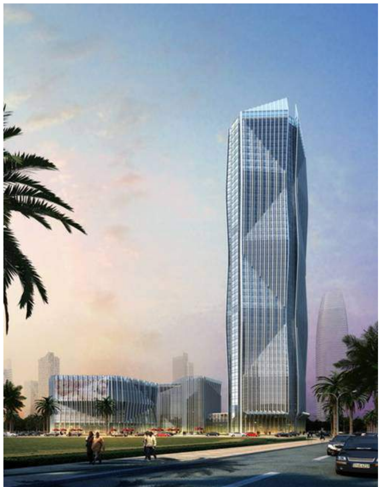
The future CBE headquarters
