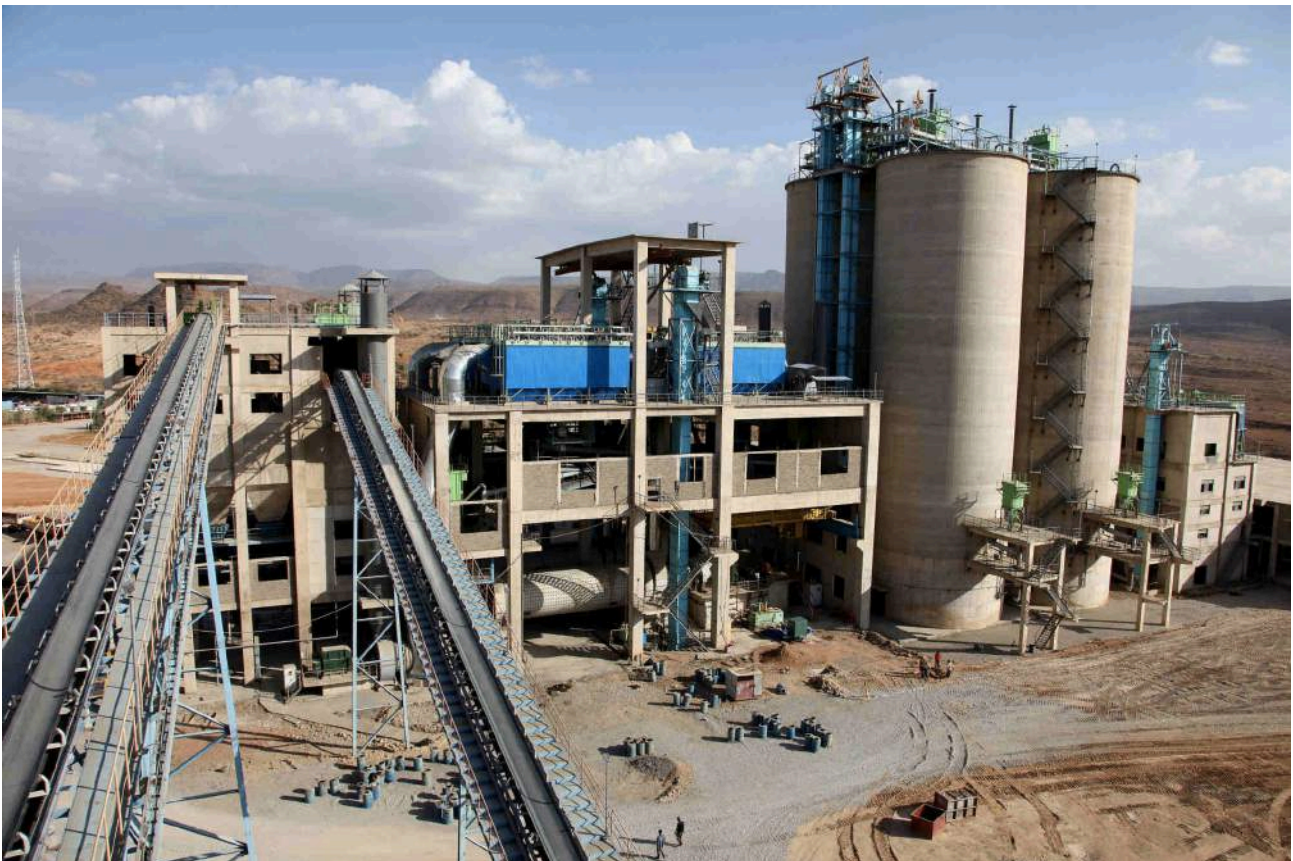
The National Cement Share Company of Ethiopia's new plant in Dire Dawa. Picture © DFID
