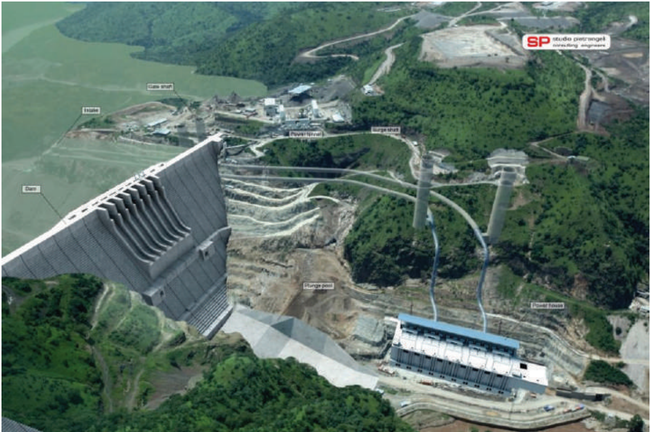
Gilgel Gibe III dam. Picture © http://www.pietrangeli.com
